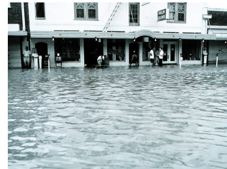
Damage and Flooding in Brownsville, Texas from Hurricane Beulah.
